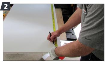
Measure the width of each panel frame and cut the panels to the proper size.
