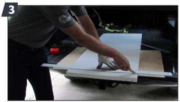
Measure the height of each panel frame and cut the panels to the proper size.
